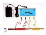
Step 3 - Plug in the power unit provided to a nearby electricity supply. Switch on at the supply and check that all the lights on the Eddy unit are illuminated. That's it . . . . . Easy!
