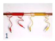
Step 1 - Wind two coils of wire (supplied) onto your incoming cold water supply pipe. It does not matter if the pipe is horizontal or vertical, or which way the water flows through the coils.
